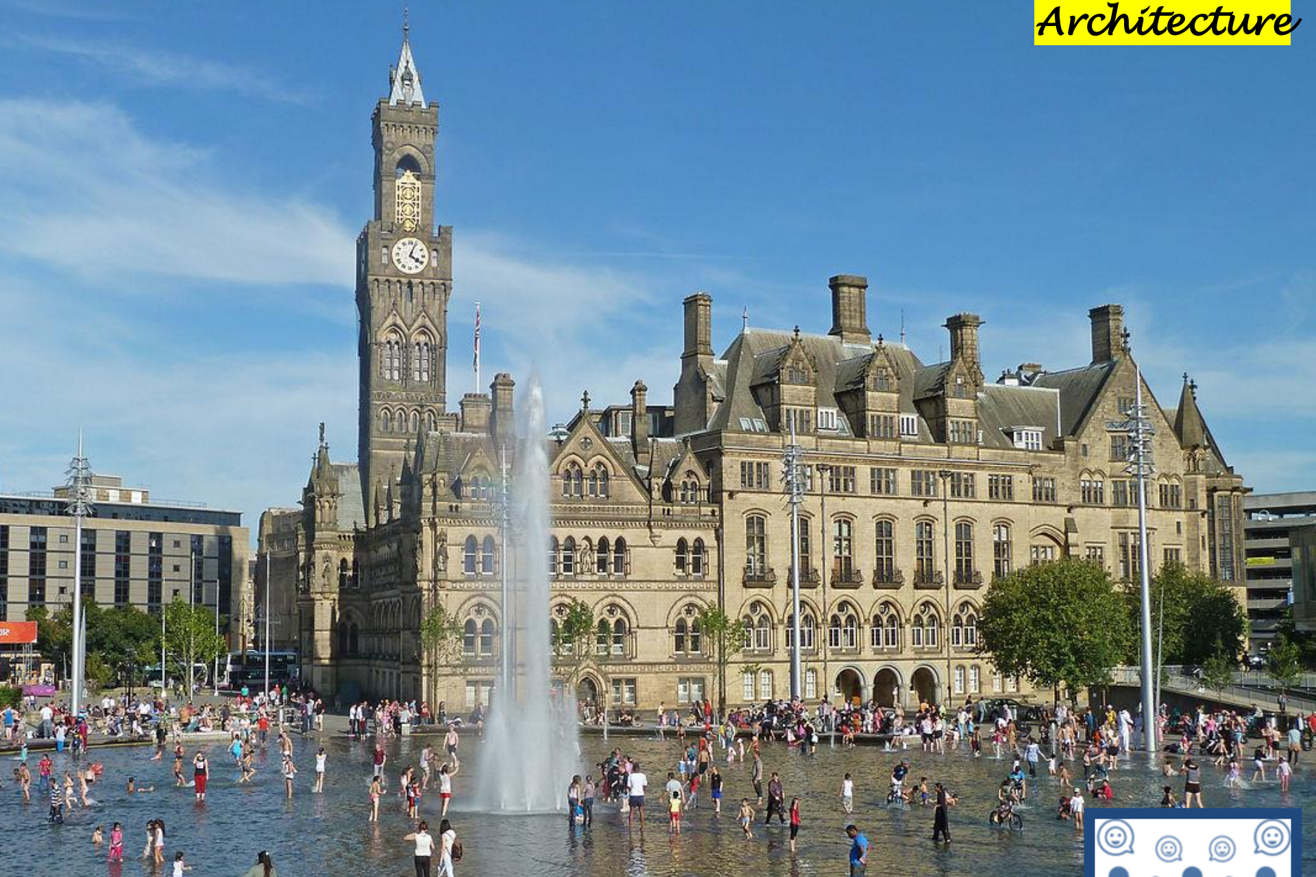
Bradford City Hall – built to replace a neo-classical building in the 1870s
